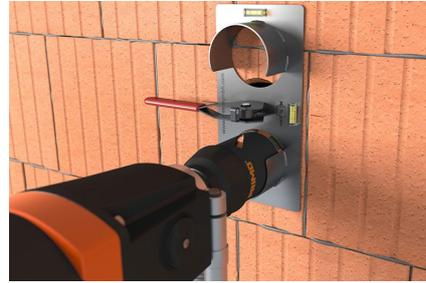
If necessary, drill additional holes. To do this, insert the drilling template and fasten and align it using the template lever with quick-clamping function.
